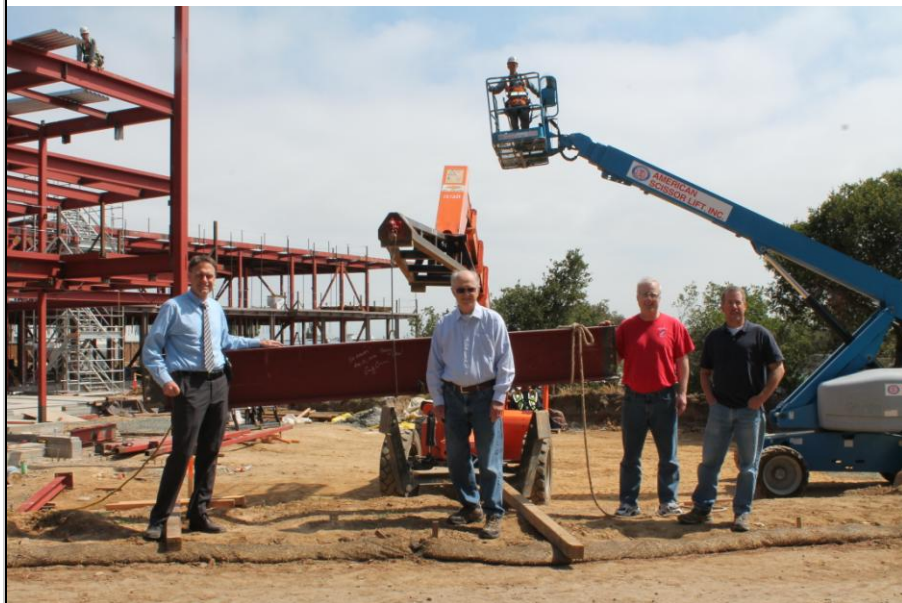
Principal Jeff Gilbert at the Ceremonial Signing of the Last Beam
